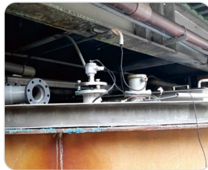
Copper sulfate storage tank
