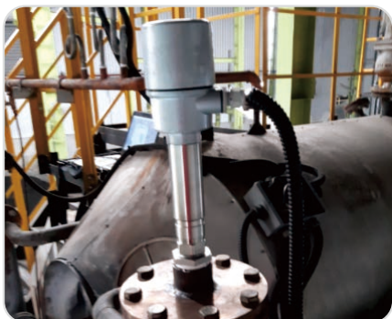
High temperature boiler
